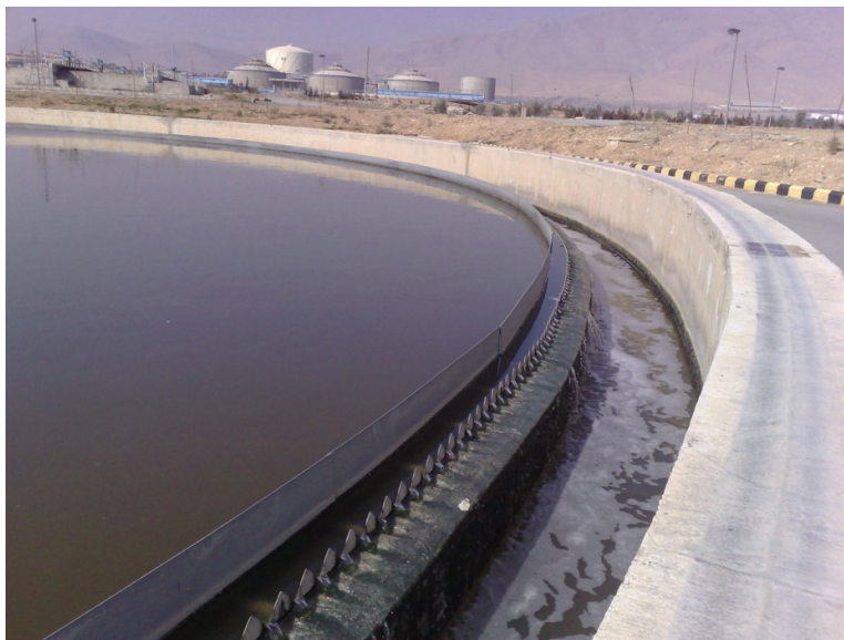
The new wastewater treatment plant of Adra
