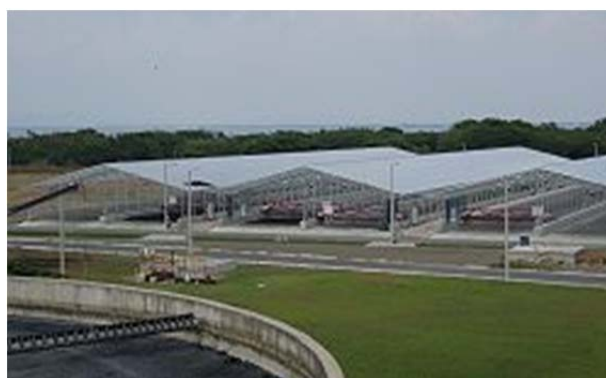
Figure 11 Thermo-System installed in Okeechobee, Florida, USA ( www.parkson.com )
